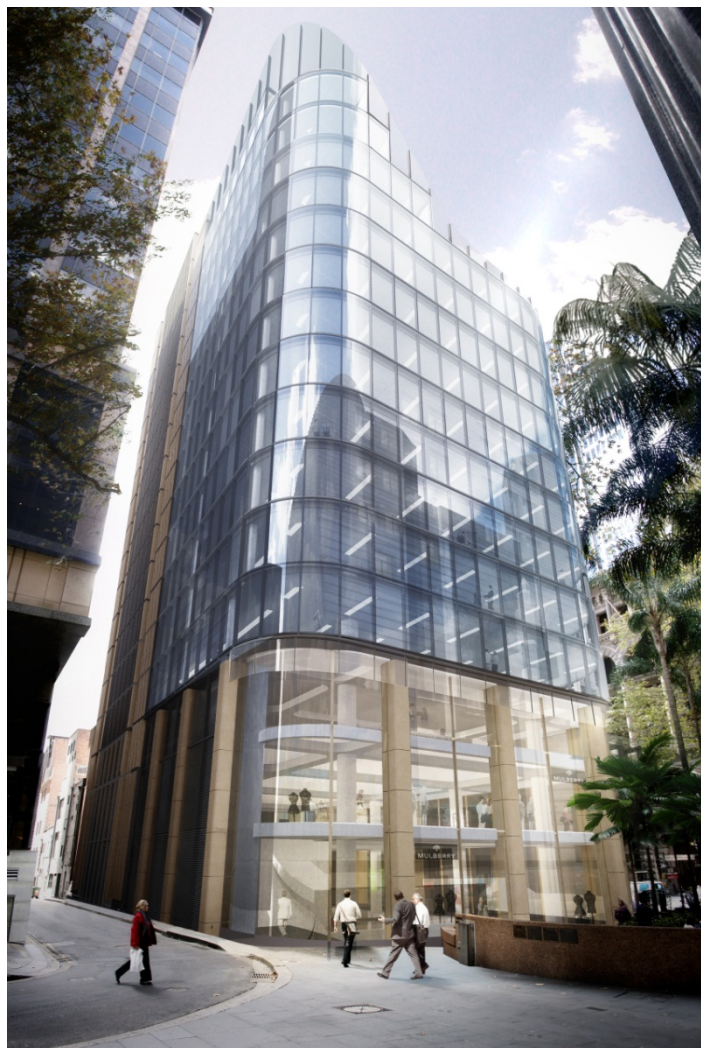
Figure 13: View of revised concept (16 November 2012 view from Wynyard Lane (with increased height of podium base and exposed sandstone columns)
