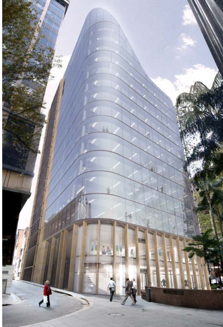
Figure 5: View of amended proposal (11 October 2012 view from Wynyard Lane (with vertical sandstone fins))
