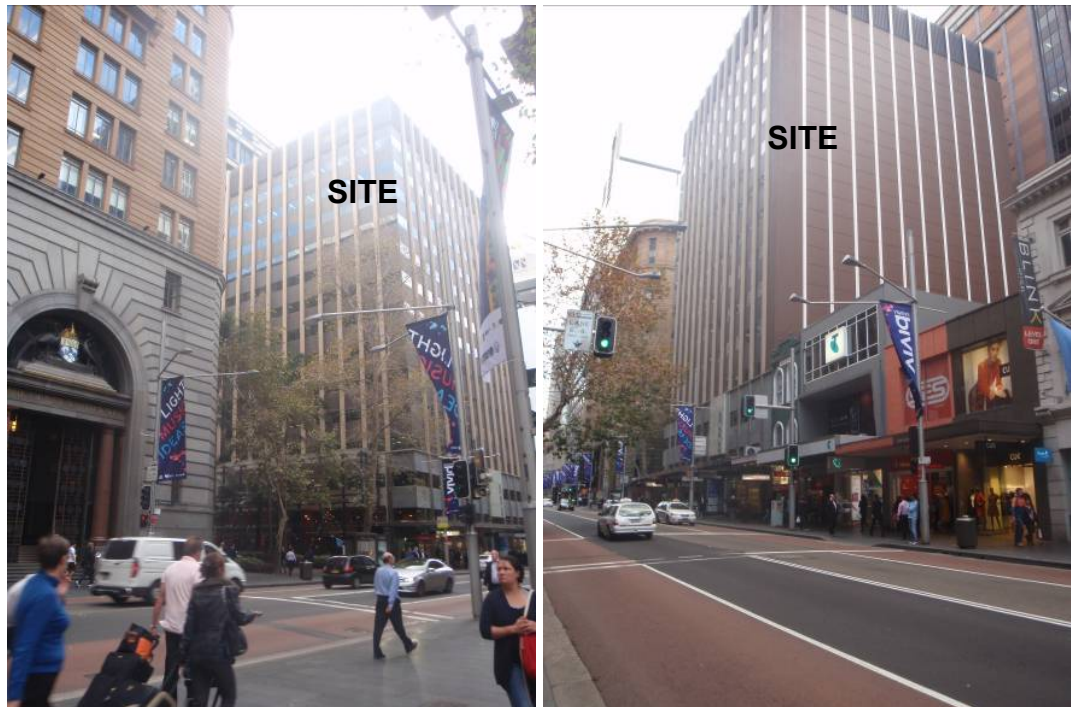
Figure 2: view of existing building from George Street
